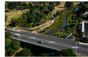
Cascades Road bridge showing the walkway connection down to the Cascades Walkway.
