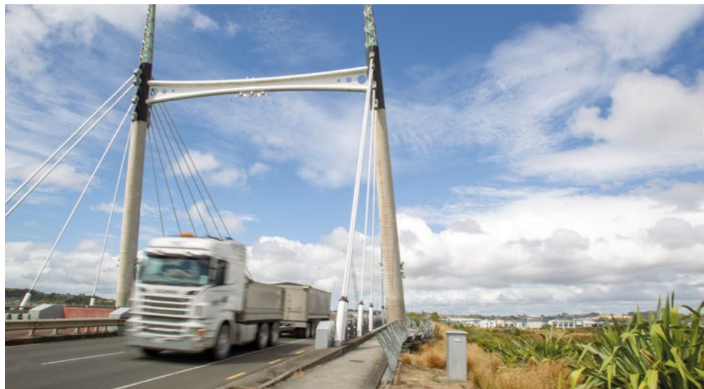
Te Uho Nikau Bridge, Flat Bush.
